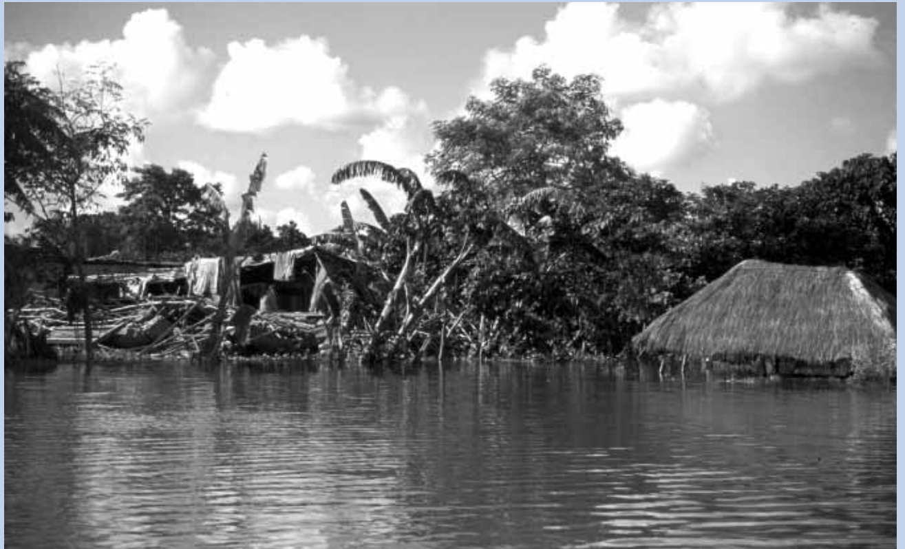
Flood damage in Bangladesh (Photo: ITDG/Janet Boston)
