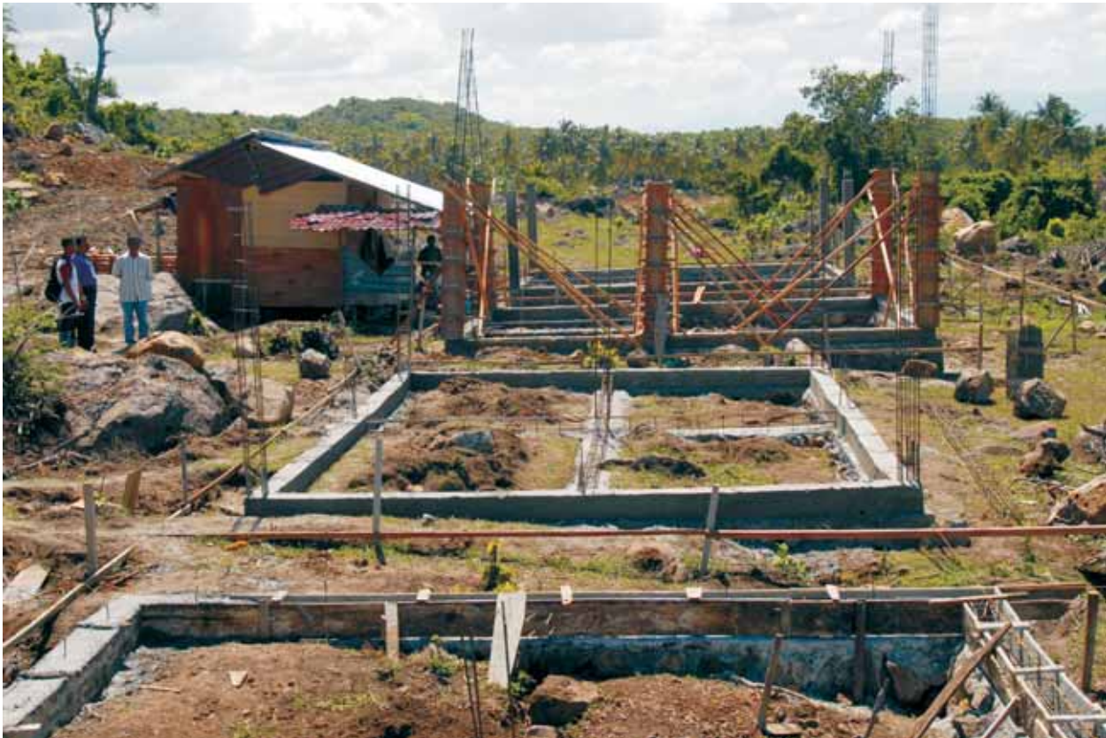
Construction in a UNEP eco-housing demonstration project, Labuye, Banda Aceh.
